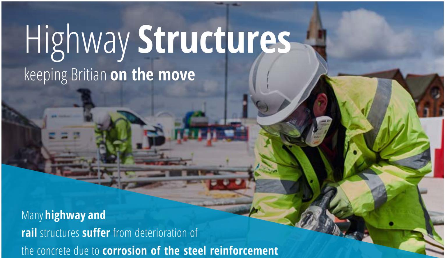
Many **highway and rail** structures **suffer** from deterioration of the concrete due to **corrosion of the steel reinforcement** which is initiated by high chloride ion levels in the concrete from de-icing salts.
