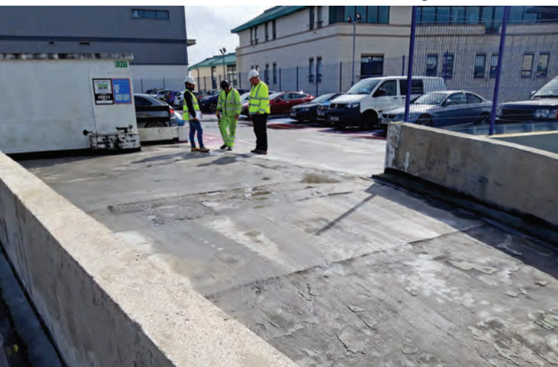
Examination of original deck.
