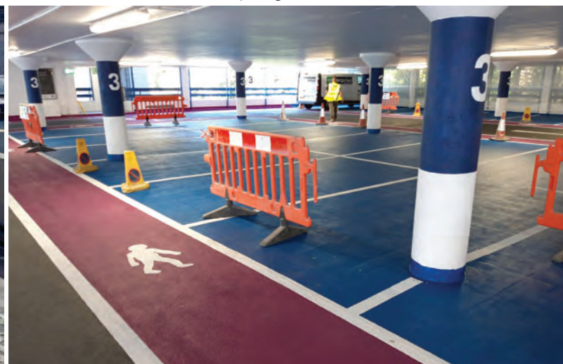
Preparing for handover of another level.
