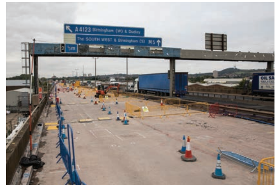
Fig. 3: Elevated sections of the motorway with expansion joints over the bents
