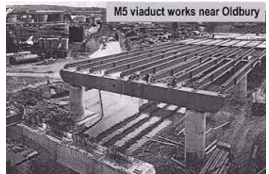
Fig. 2: Elevated construction of M5 viaduct works near Oldbury
