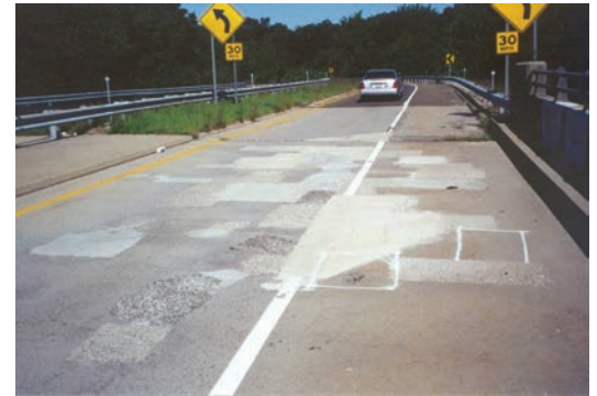
Fig. 10: Example of incipient anode formation
