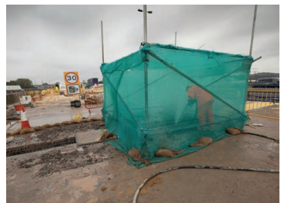
Fig. 5: Hydrodemolition of the concrete
