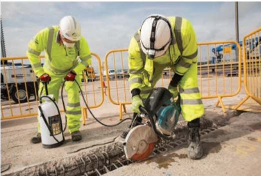
Fig. 7: Saw-cutting edges for concrete repair
