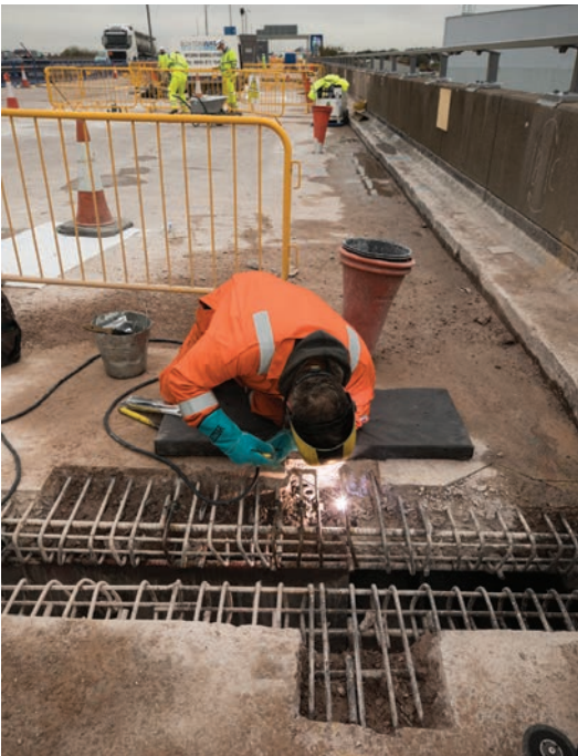
Fig. 8: Welding in new reinforcement steel
