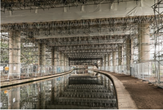
Fig. 6: Concrete repairs and installation of cathodic protection on the underside of the viaduct
