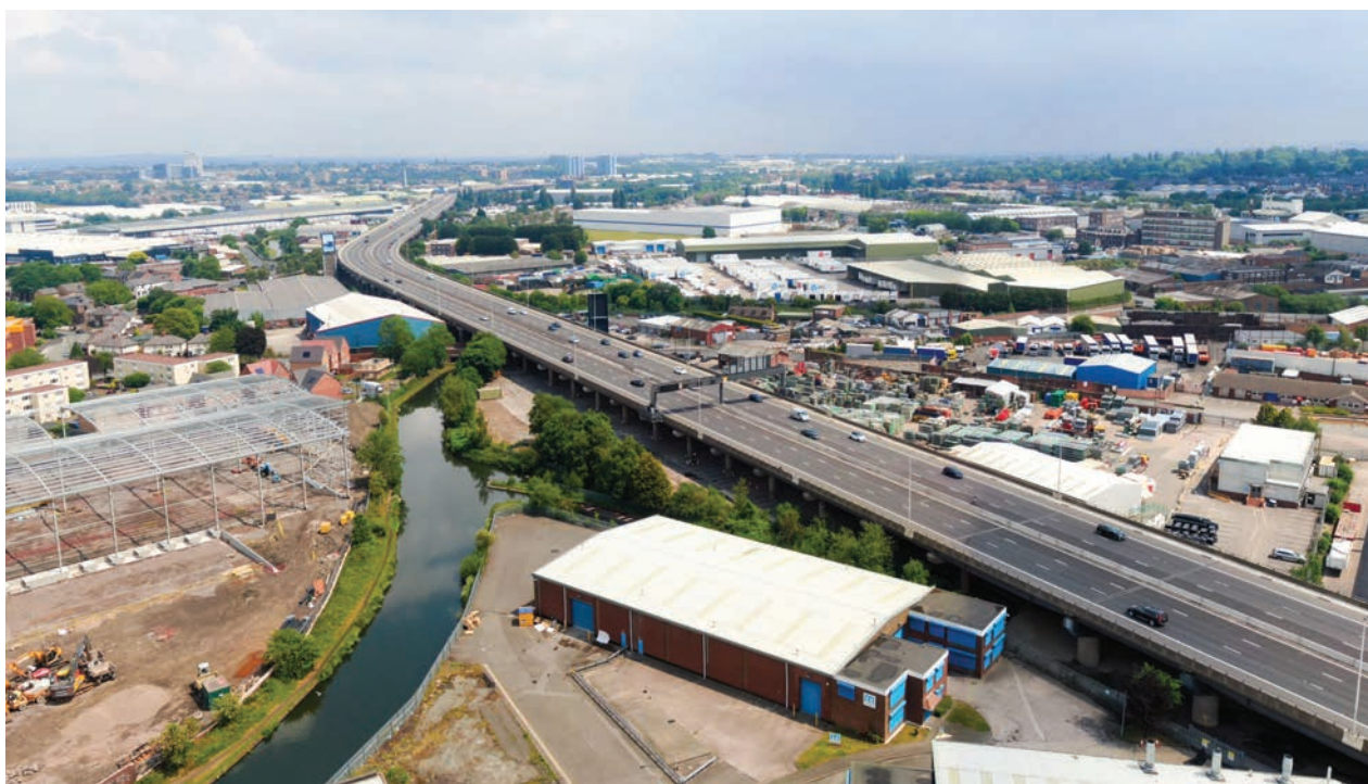
Fig. 1: Overhead view of M5 Oldbury Viaduct
