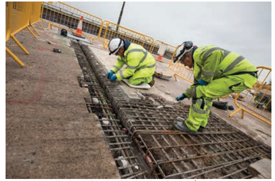
Fig. 9: Installation of embedded galvanic anodes
