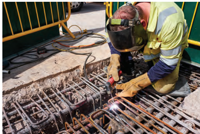
Welding in replacement reinforcing bars.
