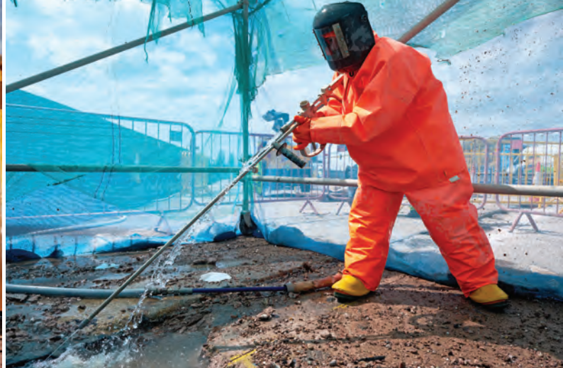
Hydro-demolition within the 3 x 3m enclosure.
