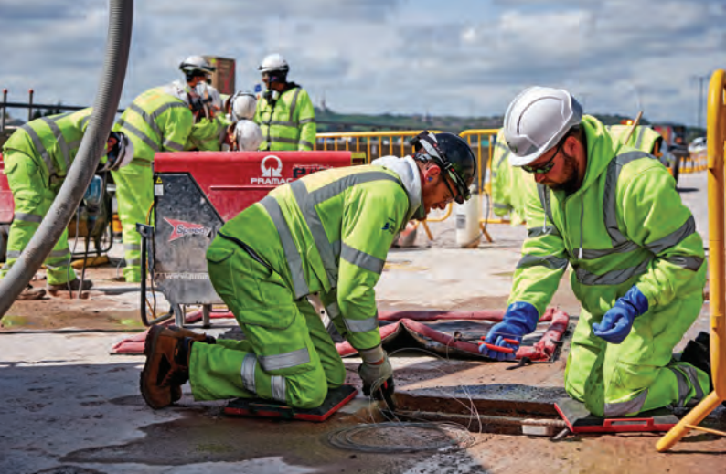
CRL's cathodic protection supervisor training an operative to install the anodes.
