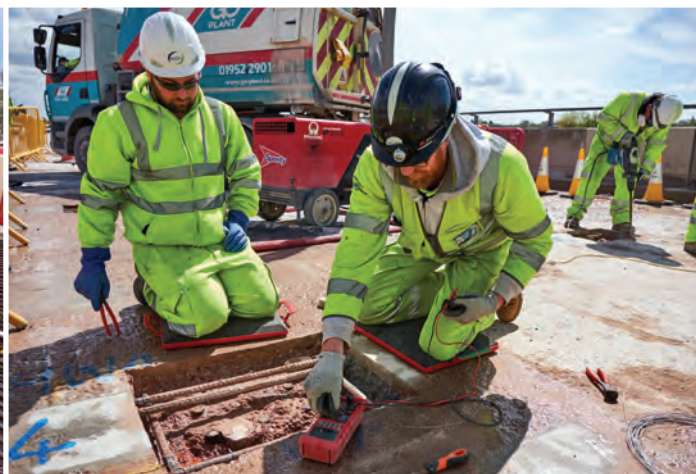
CRL's cathodic protection supervisor training an operative to carry out the continuity testing.
