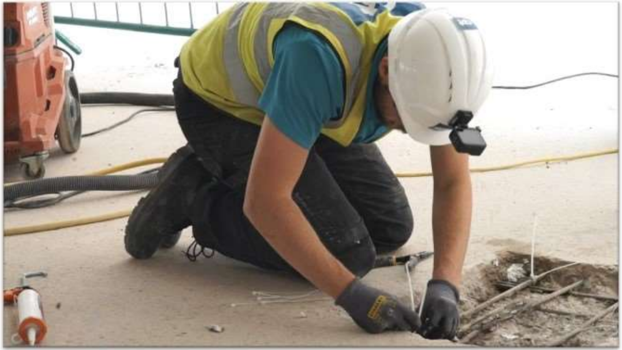
PatchGuard anode installation © CPT
