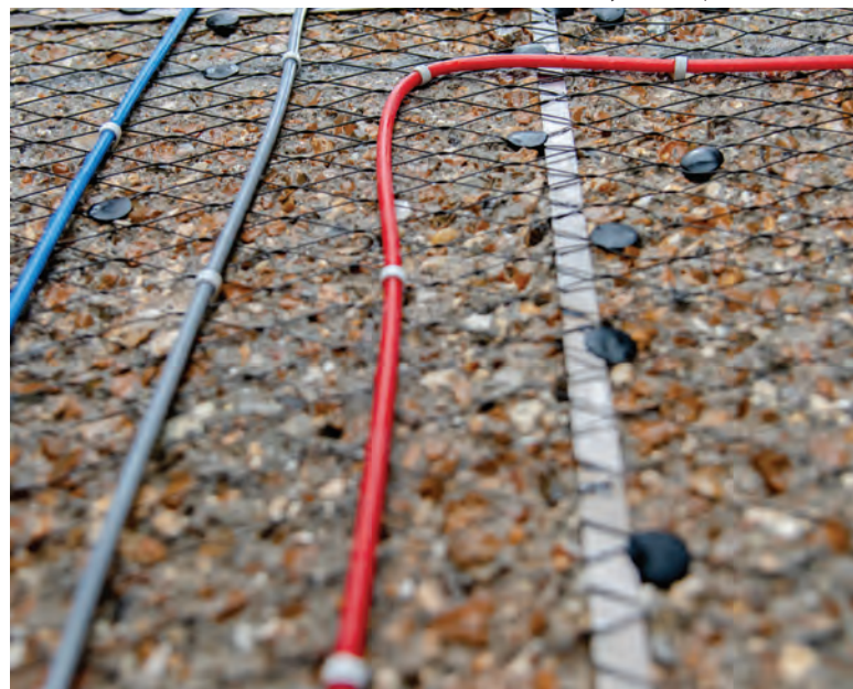
CP mesh overlay on leaf pier.
