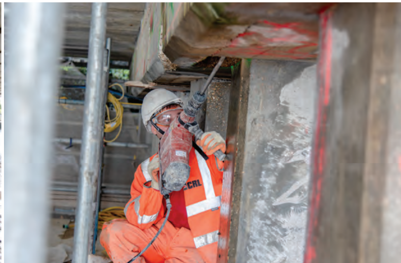
CRL breaking out repairs on bent.
