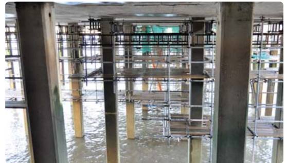
Figure 9 above: Clearing up debris after hydro-demolition and before tide rises.
