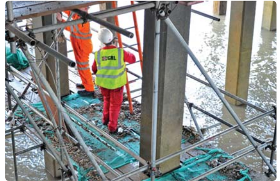
Figure 9 above: Clearing up debris after hydro-demolition and before tide rises.
